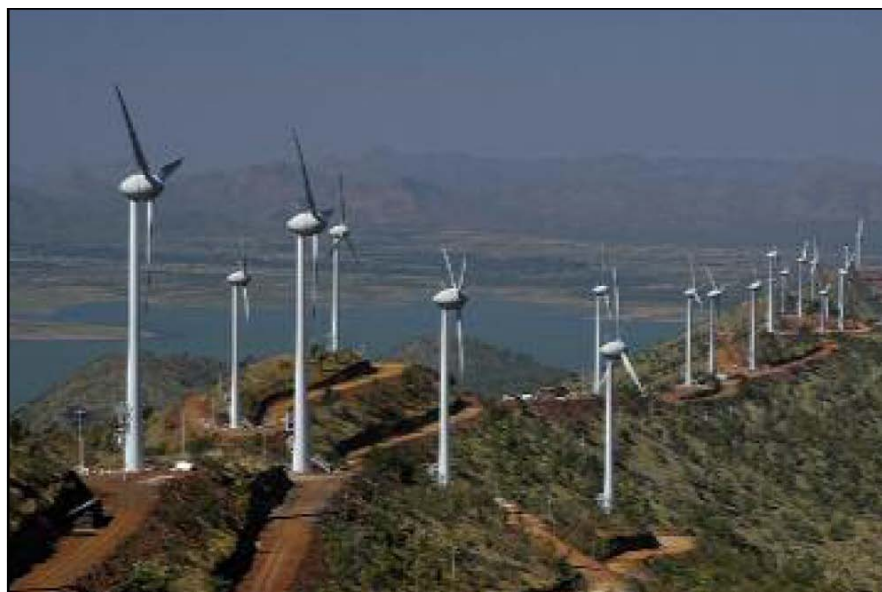
4.2 MW Wind Farm Project set up in Chitradurga District, Karnataka
